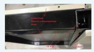
Galvanized Steel Folded to be panel. Then put lead sheet in the middle of panel, use galvanized steel strips to fix the panel. Outside face is also galvanized steel material with special painted
